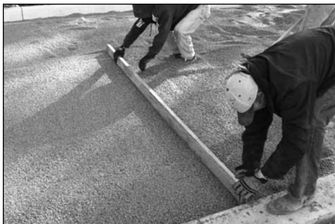
Manually screeding the No. 8 stone setting bed.
