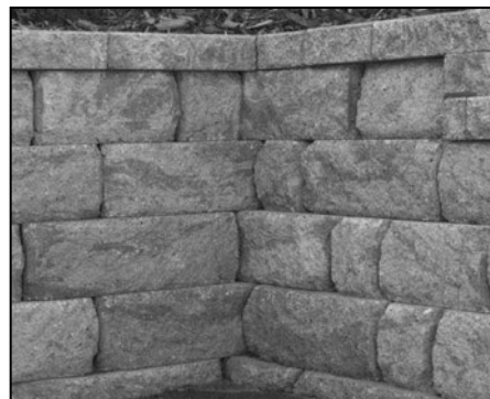
Example Inside 90-Degree Corner
