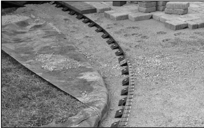
Install edge restraints.
